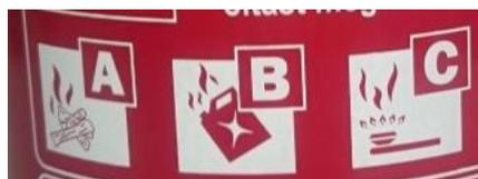
**Figure 2** Pictograms on an ABC powder extinguisher
