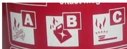
Figure 2 Pictograms on an ABC powder extinguisher
